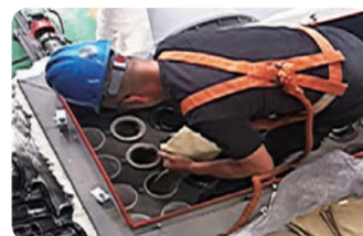
Inside bag installation
