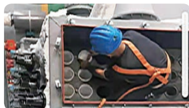
Outer bag installation
