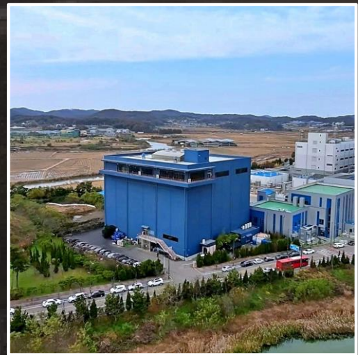
Factory 2 | Core Membrane Technology & Hollow Fiber Production
