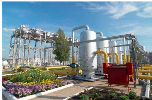
COMPRESSED AIR FILTRATION
