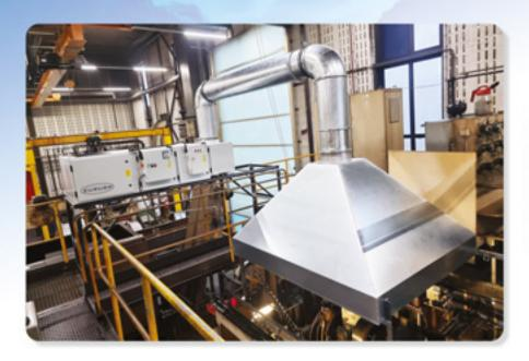
**EURUS ESP**'s can help to protect employees health by removing dangerous airborne contaminants that can cause respiratory problems. These powerful units eliminate dirty airborne particles before they settle on floors, land on expensive machinery or are inhaledsituations that can lead to accidents, workers compensation claims, Health & Safety compliance violations and expensive machine repairs.
