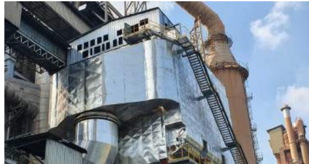
Figure 1 top view of Fabric Filter in Tasek corporation, Malaysia
