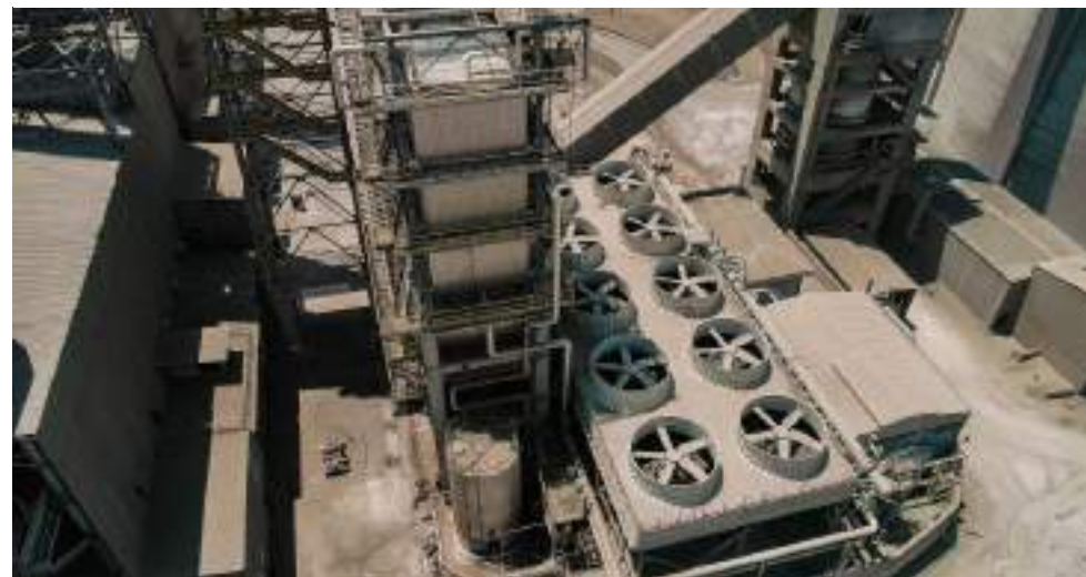
Figure 1 top view of air coolers and boiler in Narli cement factory, Turkey
