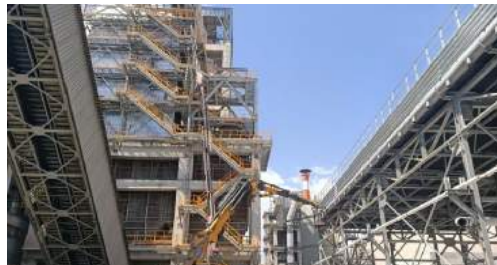
Figure 1 view of heat recovery boiler & air coolers in Sonmez cement factory, Turkey
