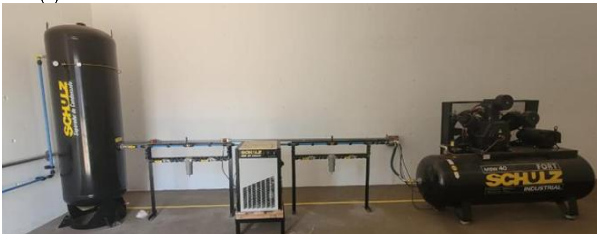
Figure 1 - Compressed air generation system (a) and separation unit (b). (Authors, 2026).
