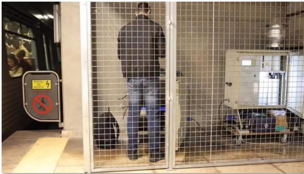
Figure 2 – Placement of scientific grade instruments at the end of the platform.
